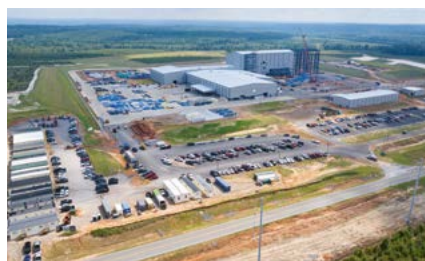
Aurubis, USA: The first multi-metal recycling plant in the US
