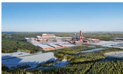
Stegra, Sweden: The world's first 100% hydrogen-based steel plant
