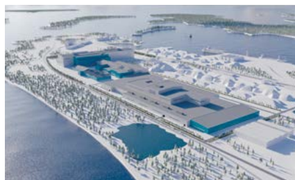
SSAB Lulea, Sweden: Sustainable cold rolling and strip processing complex
