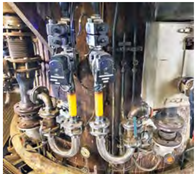
Gas supply line with new control and shutoff assemblies.
