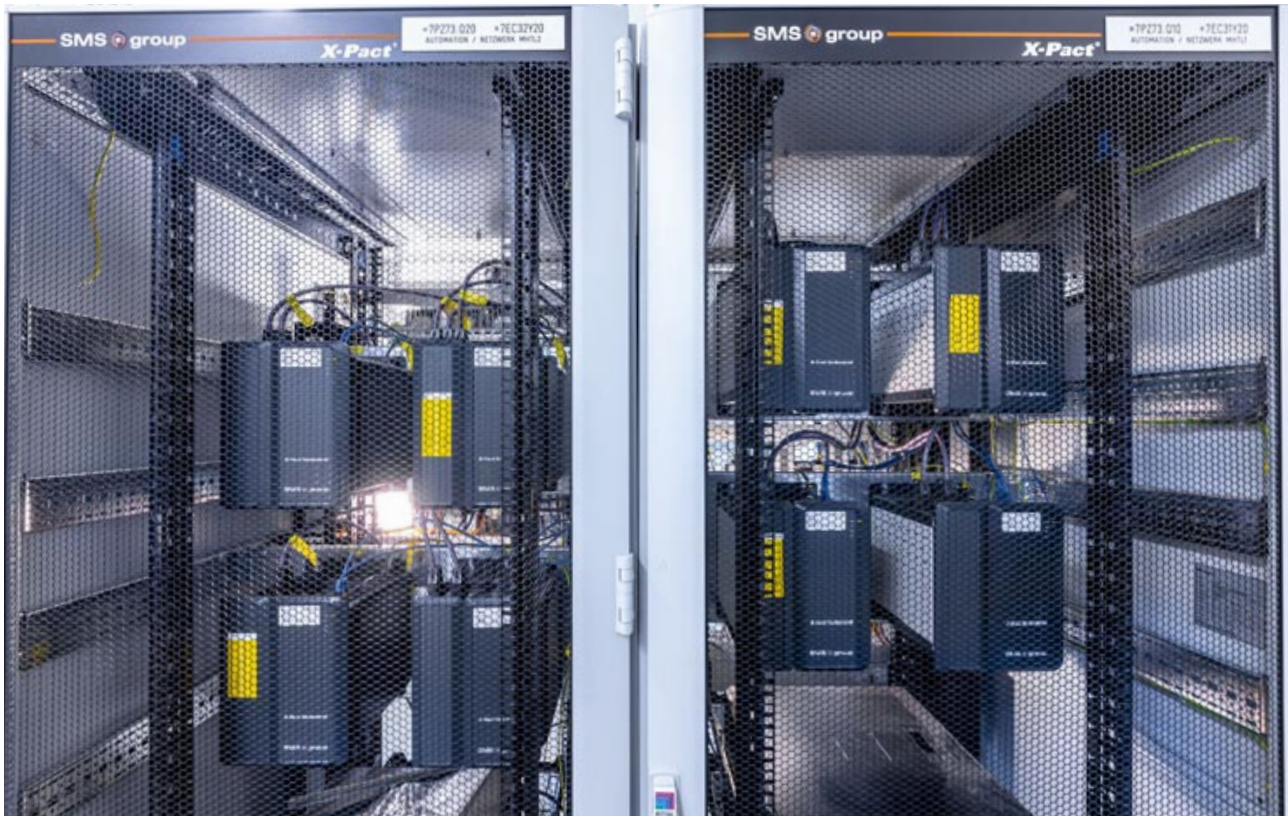
X-Pact® automation cabinet with 8 real-time control systems for the plant automation.
