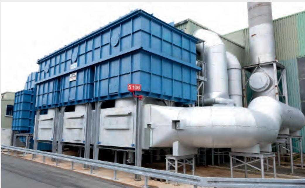
*A regenerative incineration system (here with three chambers) burns the solvent-containing air and regains the energy produced.*
