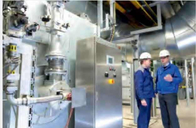
*For some products, the hardening oven can be fueled completely by the energy reused from the evaporated solvents.*
