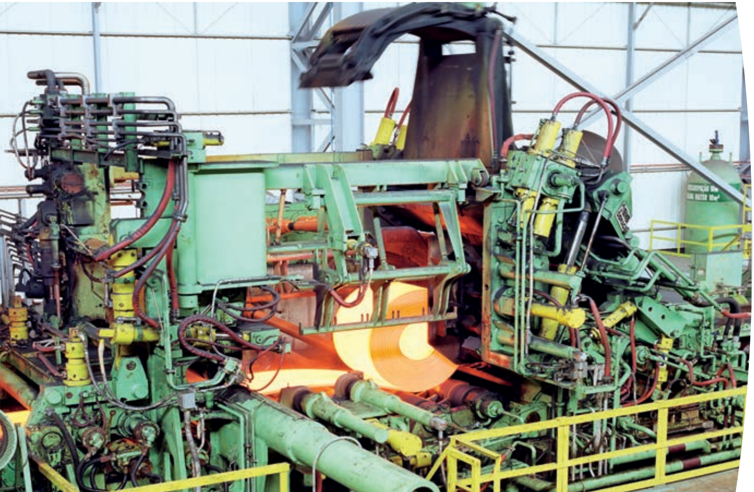
Installation of a coilbox in the second modernization stage.
