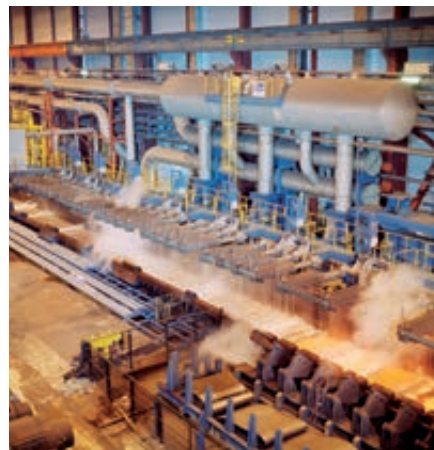
Laminar cooling section.
