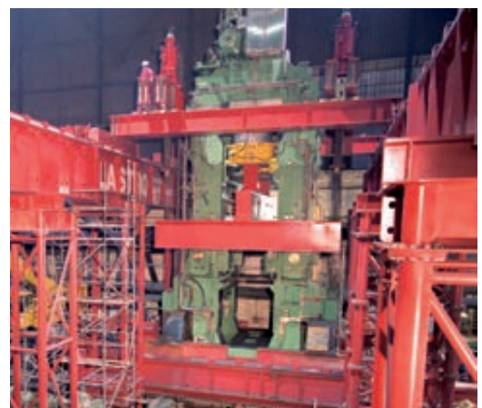
The new roughing stand is pushed into the rolling line.
