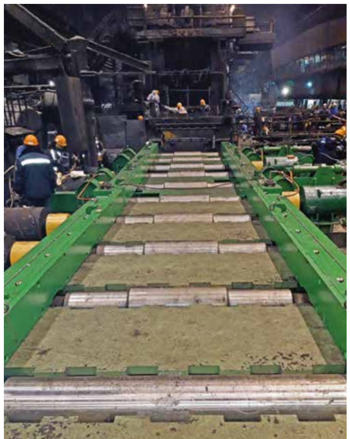
Conversion phase in the shear area. Installation of a new hydraulic side guide from SMS group.
