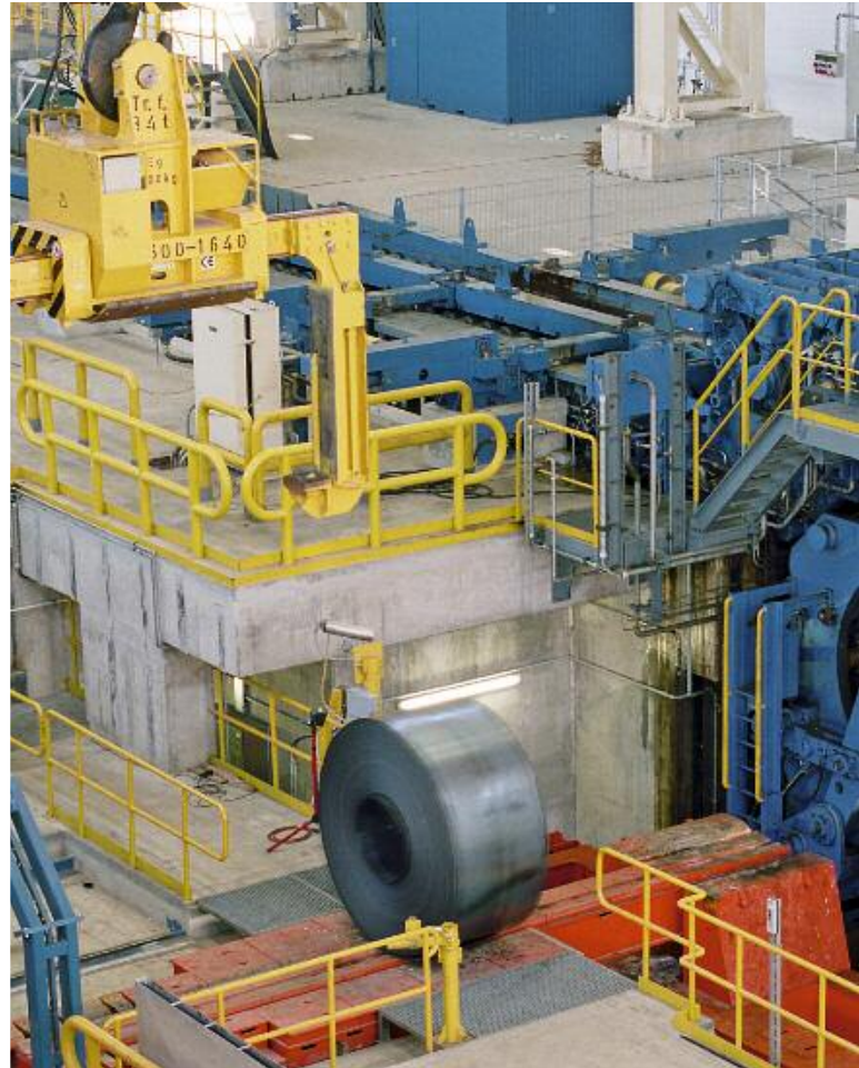
Three-roll coiler with Step Control.
