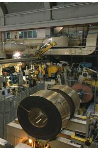
Under work rolls and Level 2 automation operated by KME Italy.
