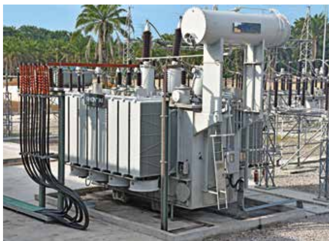
One of the two 132/33kV step-down transformers of 150 MVA rated capacity with primary taps for secondary voltage regulation. The transformers were sourced by SMS group China.
